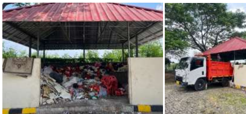
Fig. 5: Temporary Waste Storage Site & Garbage Truck on Campus
