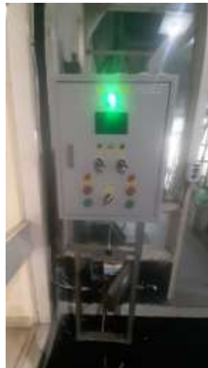
Figure 6. Impact Test Platform Altitude Control System Implementation
