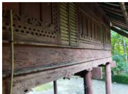
Gambar 12. Dinding Sumber: Hasil Survey, 2024
