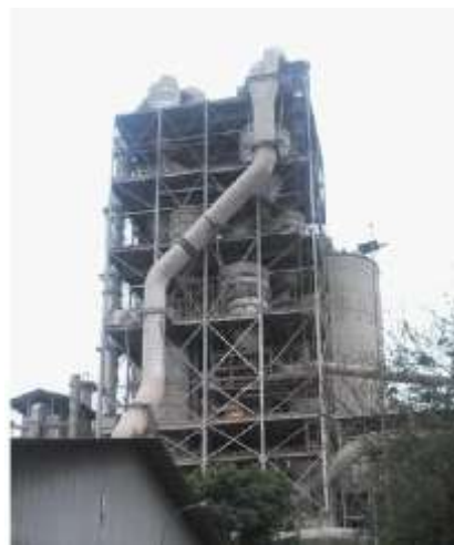
Gambar 4. Suspension preheater
