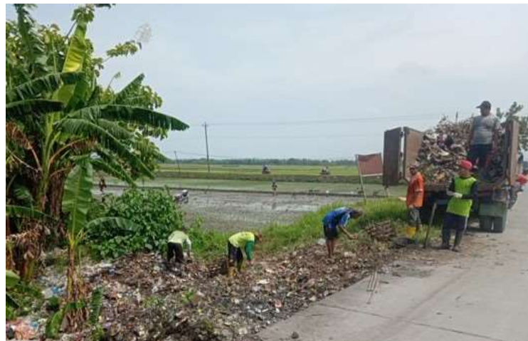
Fig 3. Post-Disaster Floods Cleaning
